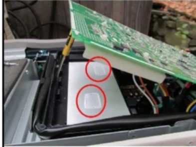
ODU main board replacement
