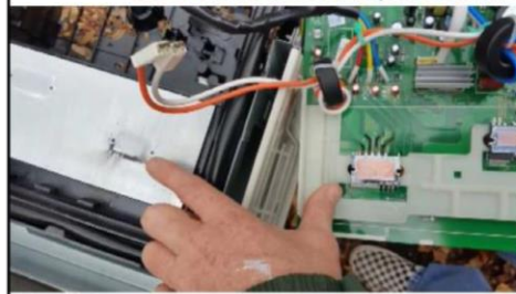
ODU main board replacement
