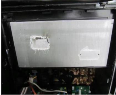
ODU main board replacement
