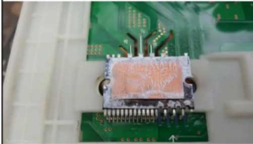
ODU main board replacement
