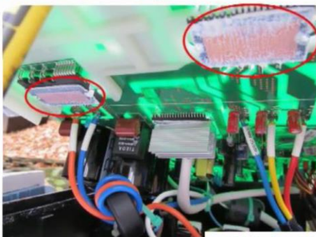
ODU main board replacement
